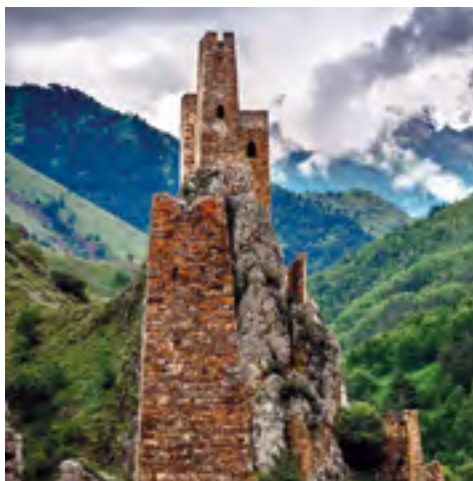
Vovnushki Tower Complex, Ingushetia
